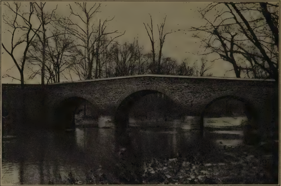
STONEY BROOK BRIDGE, PRINCETON
